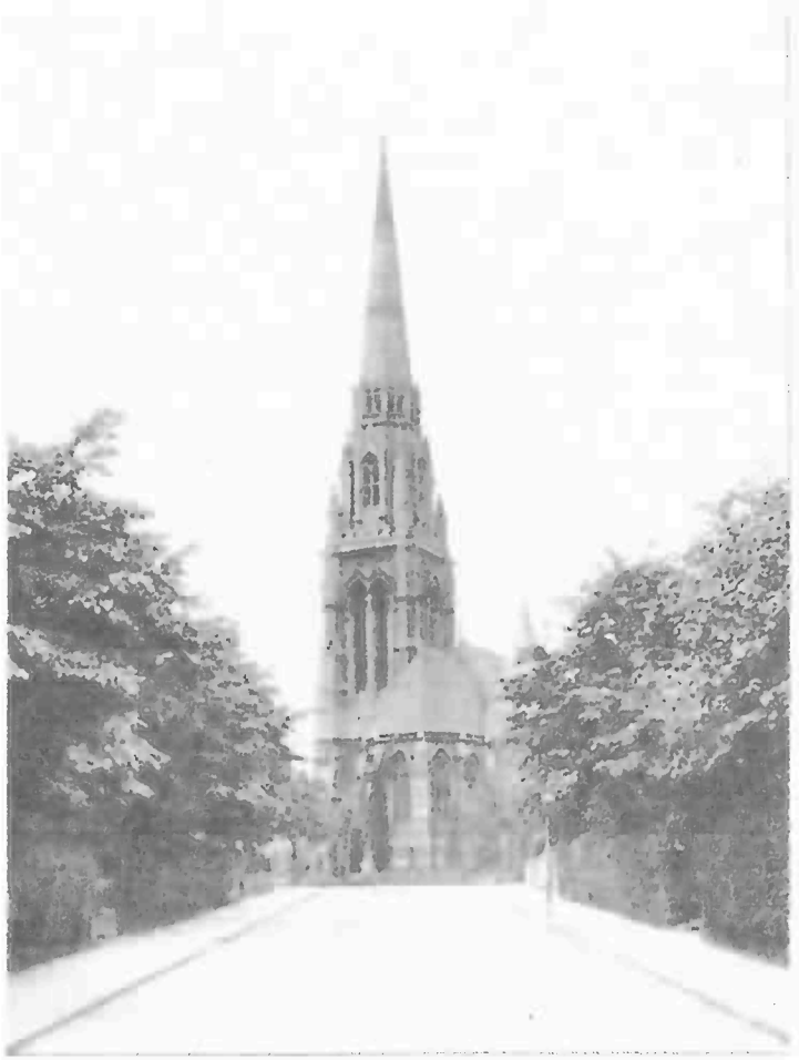
THE CHURCH FROM THE EAST.
